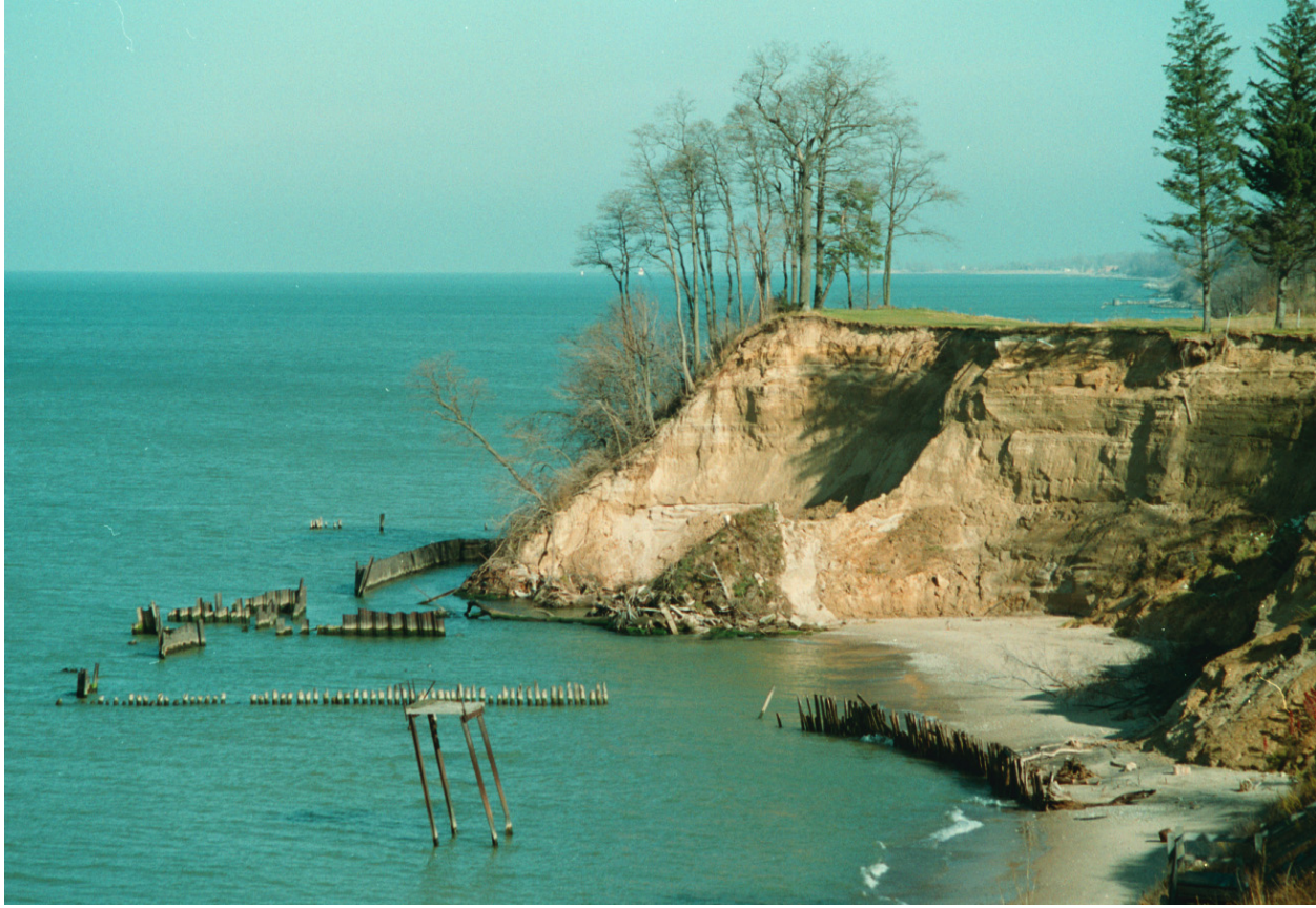
Figure IV-2-22. Lake Michigan shore south of St. Joseph, Michigan (November 1993). A triangle-shaped wedge of the bluff has recently slumped. The bluffs in this area have suffered rapid retreat, and many homes have been destroyed. At least three factors account for the erosion: (a) offshore downcutting of the till lake bottom; (b) wave attack on the bluffs; (c) ice expansion and lubrication of bedding planes caused by groundwater
