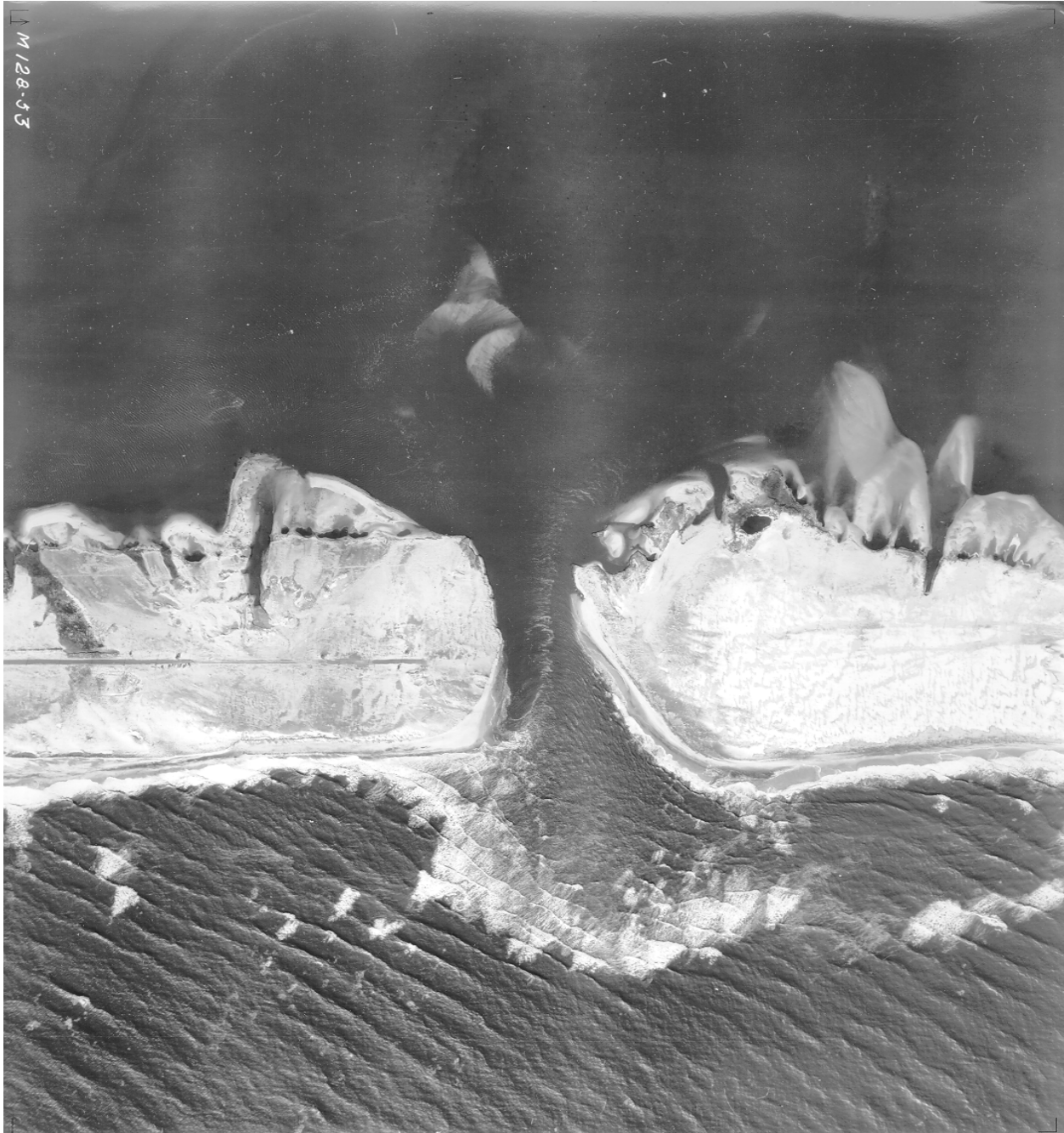
Figure IV-3-27. Shinnecock Inlet, New York, 29 November 1938, photographed only 2 months after the barrier island was breached during the Great New England Hurricane of 21 September 1938. North is to the top of the image. The body of water to the top is Shinnecock Bay, and the Atlantic Ocean is on the bottom. The inlet already displays an oval ebb-tidal shoal. A small shoal in Shinnecock Bay indicated development of a flood shoal. Washover fans, remnants of the storm, can be seen on both sides of the inlet. (Photograph from Beach Erosion Board archives)
