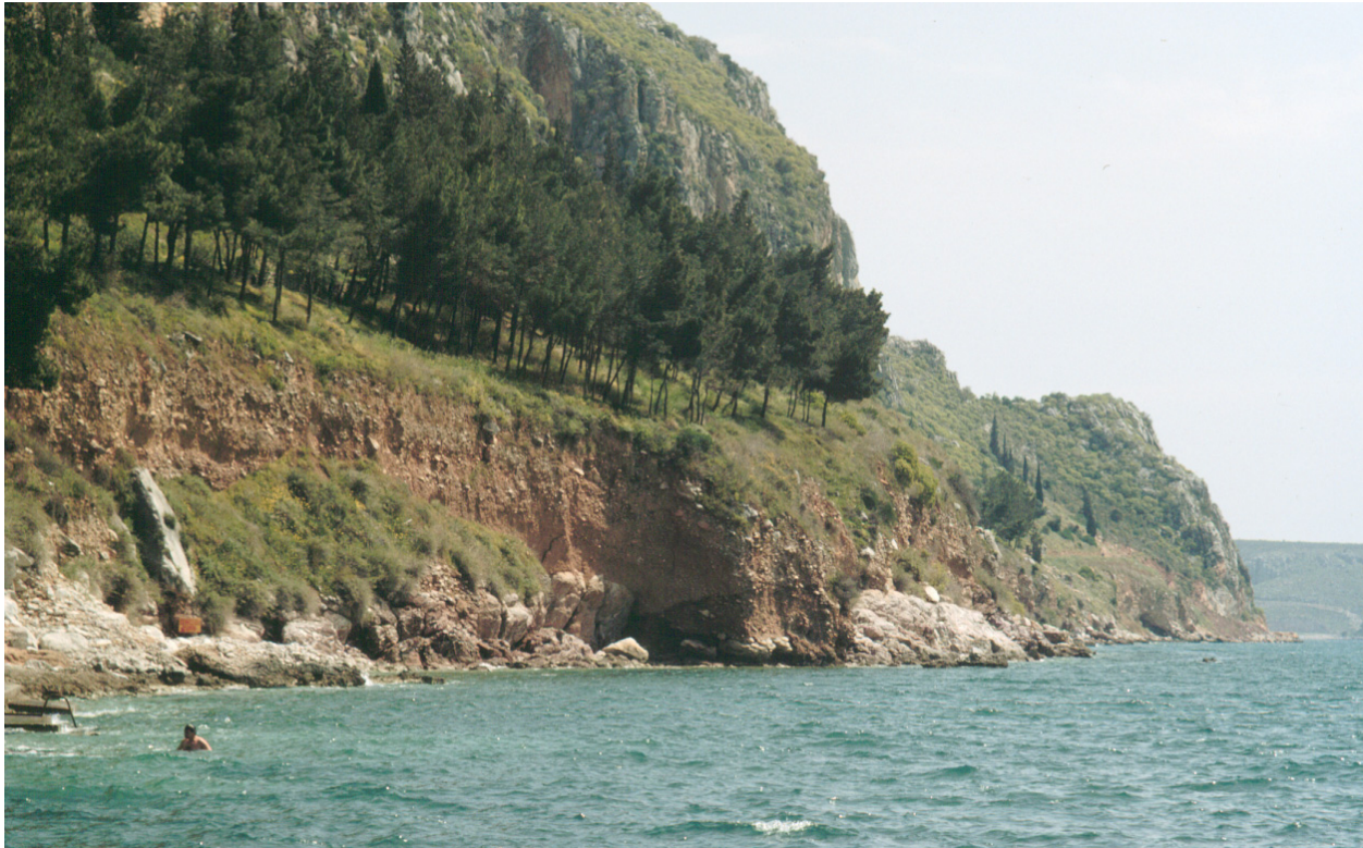
Figure IV-2-21. A section of cliff, projecting out from the shore, is likely to collapse soon. To the left, rubble at sea level marks the location of a previous slump. The lower cliffs are poorly cemented conglomerate while the higher, vertical cliffs (above the trees), are limestone (near Nauplió, Greece, April 1992)
